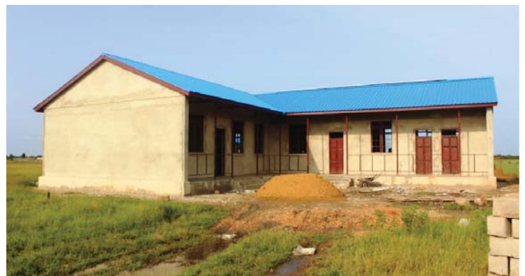
Construction of Abyei Women's Center
