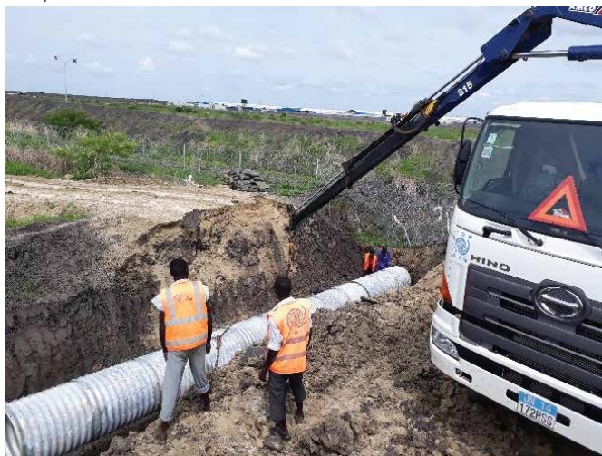
Installation of drainage culverts prior, IOM/Makhatsa 2017.
