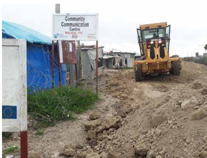
Road repair in Sector 2. IOM/Makhatsa 2017.
