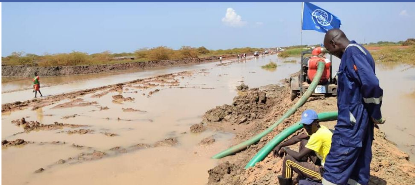
Site care and maintenance activities in Bentiu IDP site that include reclaiming the main supply road by pumping water out © IOM CCCM 2021
